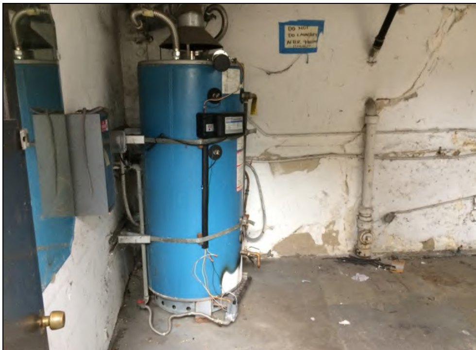
Photo 14: View of water boiler within a room, located west of the property.
